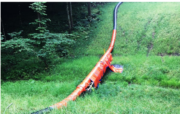
Temporary Waterline Permitting
