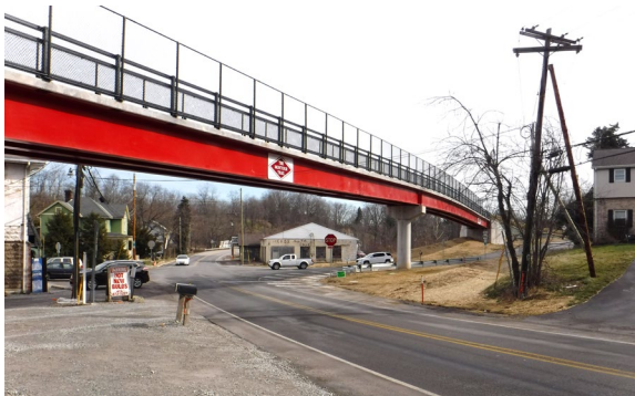
PA 980 Realignment & Pedestrian Bridge
