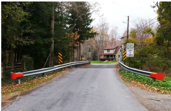
Prefabricated Superstructures – Mill Creek Bridge
