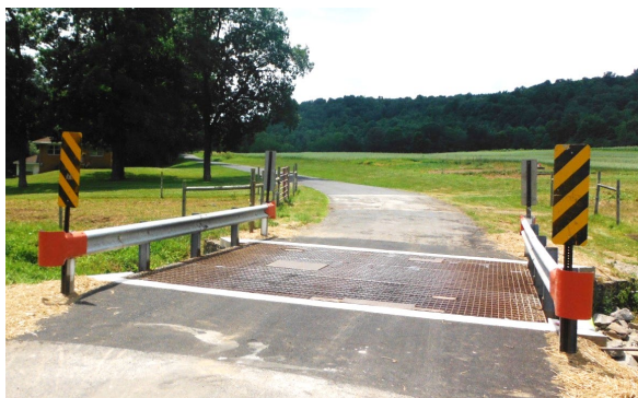
Harvey Road Rhoades Farm Bridge
