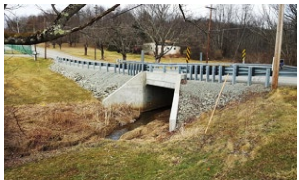
Hills Church Road Bridge
